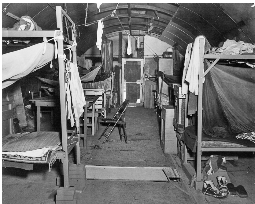
Figure 3.2. Inside a Quonset hut at Camp Roxas, 1950s. Source: Photograph courtesy of Humanities Guåhan, A Journey Home: Camp Roxas and Filipino American History in Guam , an exhibition funded by the National Endowment for the Humanities, We The People Initiative.
